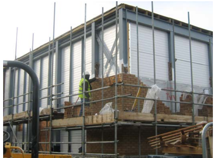
The brickwork starts to take shape around the new studio!
